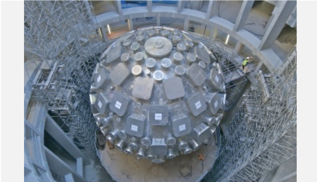
1217-01: Bordeaux. CEA's CESTA center. The Megajoule Laser's experimental chamber with its concrete shield. This sphere 10m in diameter and 10cm in width weighs 140 tons. 240 laser beams will converge on
