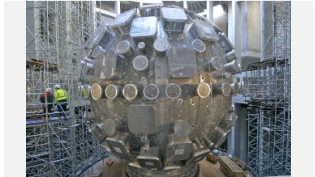
1217-02: Bordeaux. CEA's CESTA center. The Megajoule Laser's experimental chamber with its concrete shield. This sphere 10m in diameter and 10cm in width weighs 140 tons. 240 laser beams will converge
